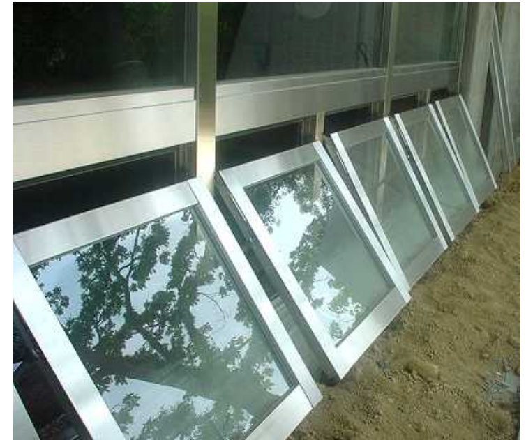
Exterior view of the lower windows for air supply (Bathhouse)
